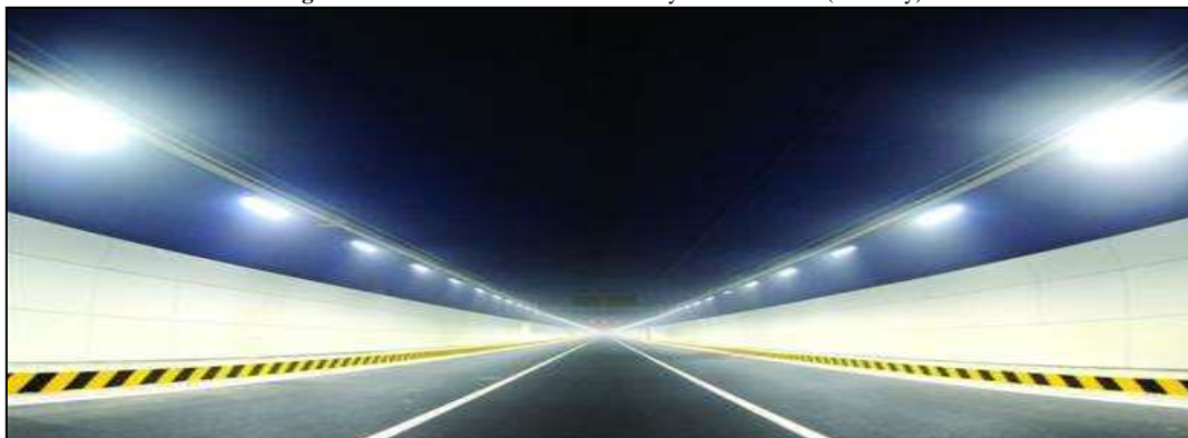
Figure-2. An Interior of the Jiaozhou Bay Subsea Tunnel(one-way)
