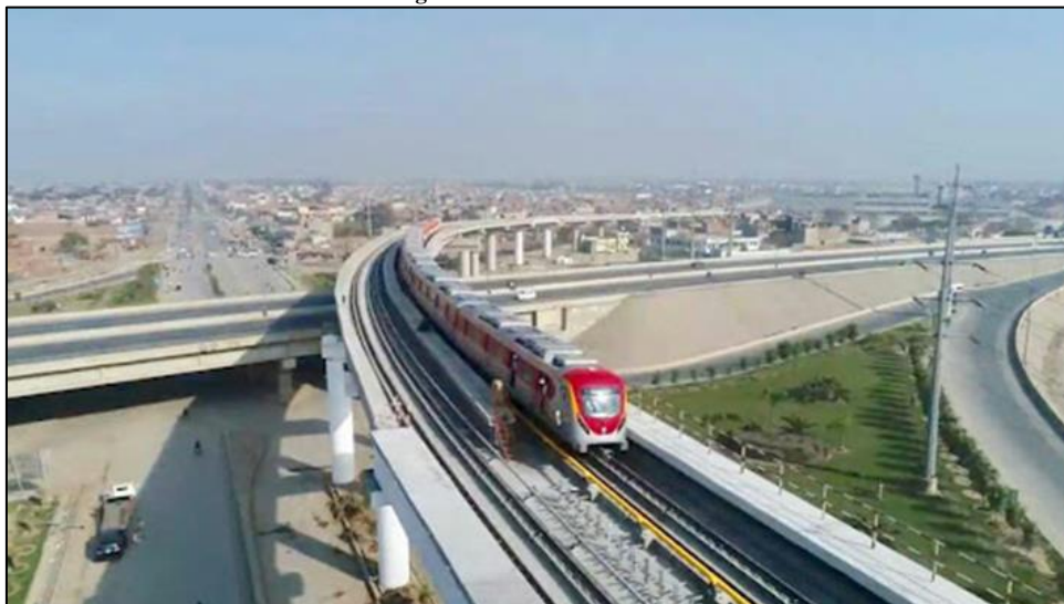
Figure-18. Tram infrastructure
