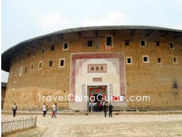
Figure-2. Outside View of Hakka Tulou
