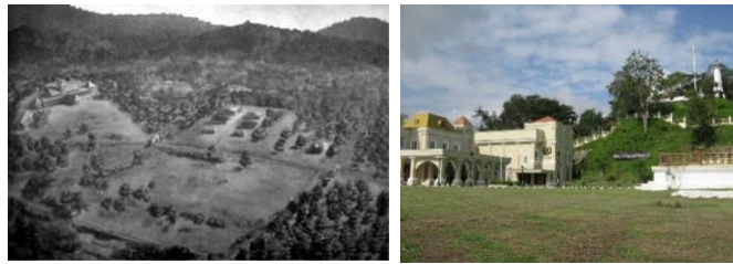
Figure-2. The illustration of the old view of Sri Menanti town (left) and the current view of Maziah Palace (right).
