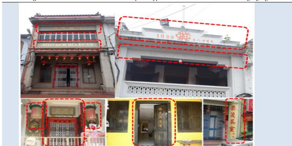
Figure-2. Red dotted line indicate an example of type and location of traditional building signage
